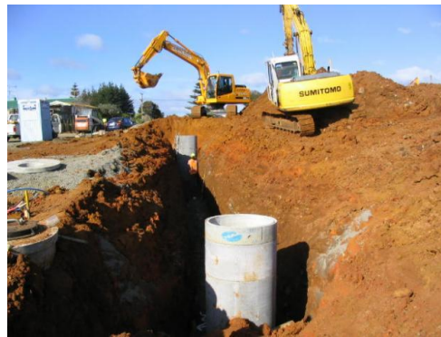
Figure 2 Excavation permit and clearances
